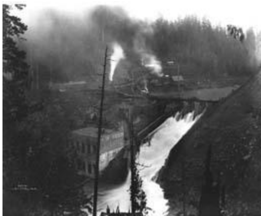
Elwha River Dam and electric power plant, 1914
